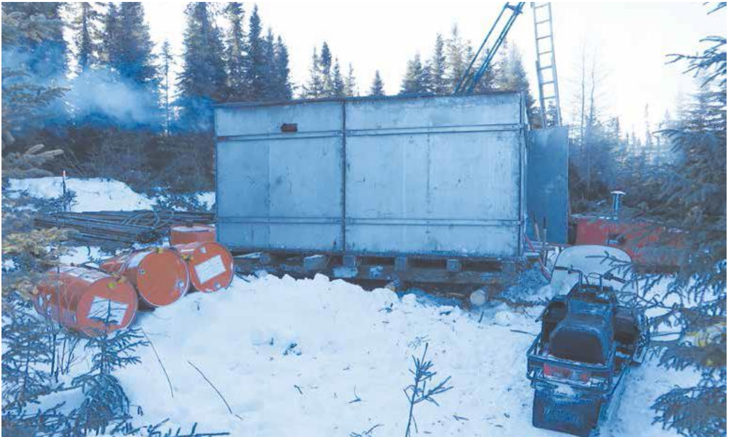
Drill rig on the first hole of the Woco Gold Vein.
